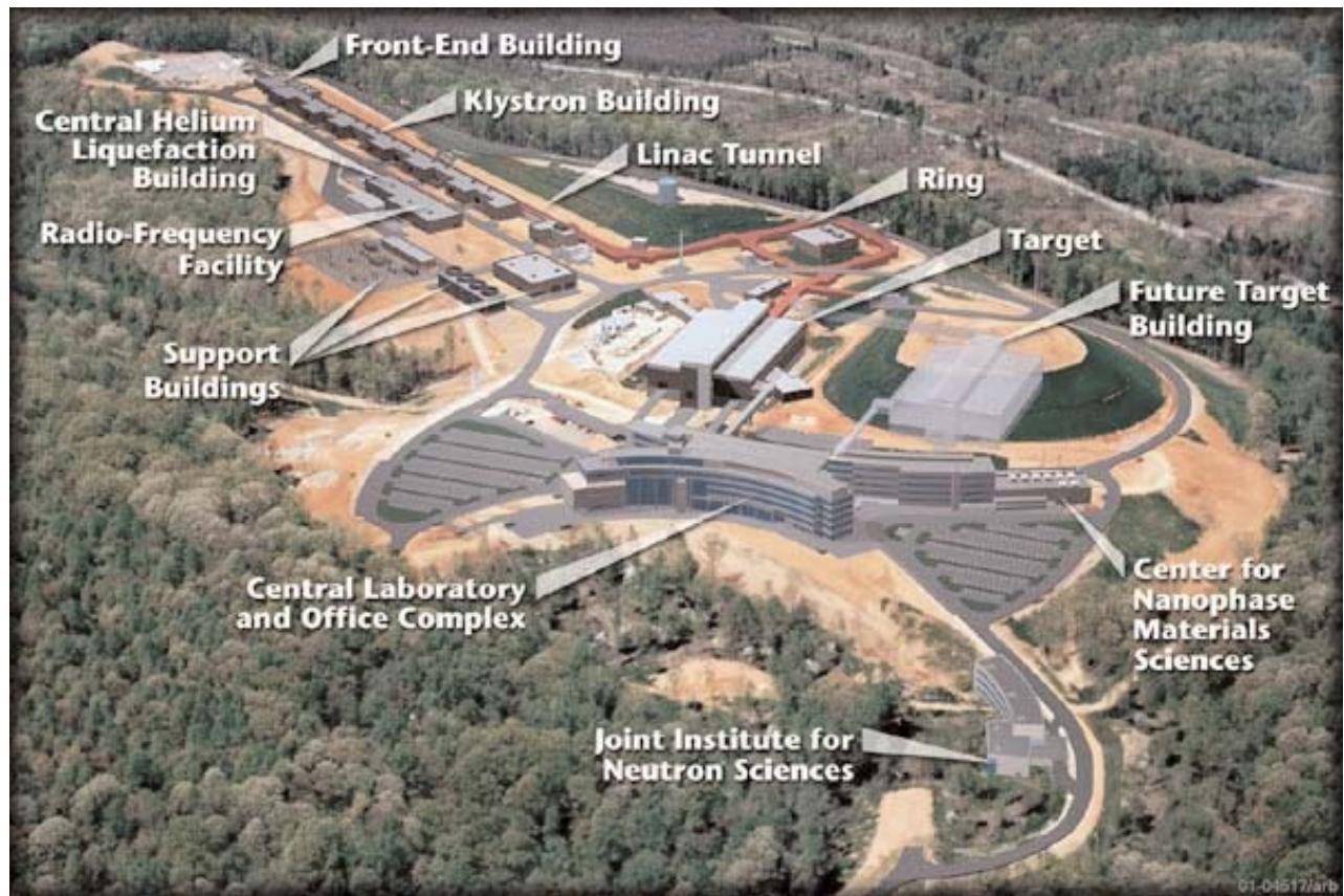
Figure A-2 Spallation Neutron Source Facility at Oak Ridge National Laboratory.
